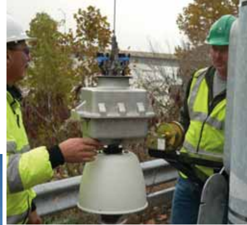
Maintenance done safely and easily at ground level.
